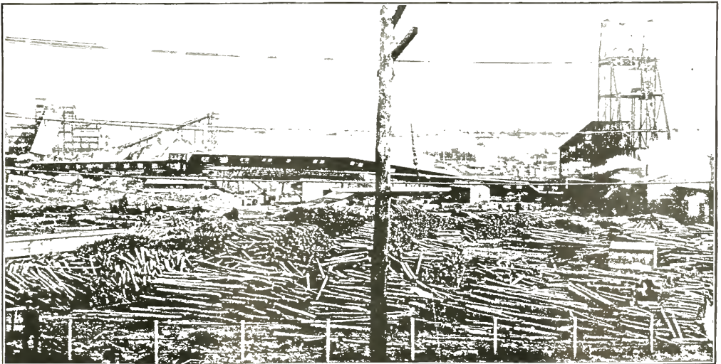
FILES OF WOOD TO BE USED IN THE MARVINE MINE OF THE HUDSON COAL CO. FOR POSTING ROOF
